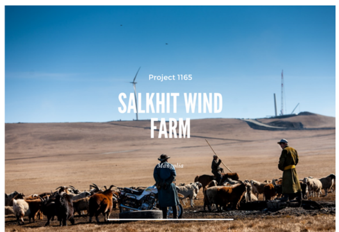
Project 1165: Salkhit Wind Farm in Mongolia
